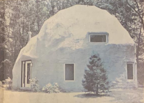
A recently completed foam home in Falls Village sits on a four-acre site and has two bedrooms, two baths and an attic area. Moore estimates a starter shell home can be put up for about $26,000, leaving the occupant to expand it when finances permit.
